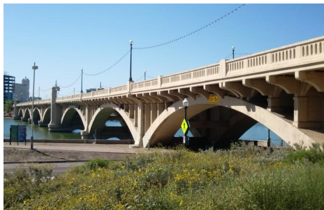
Photo courtesy of Brian Davis, Stanley Consultants
