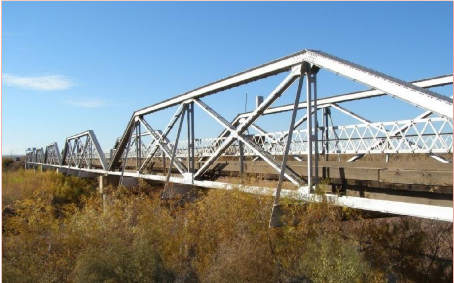
Historic 6 span pony truss bridge – posted for 8 ton live load
