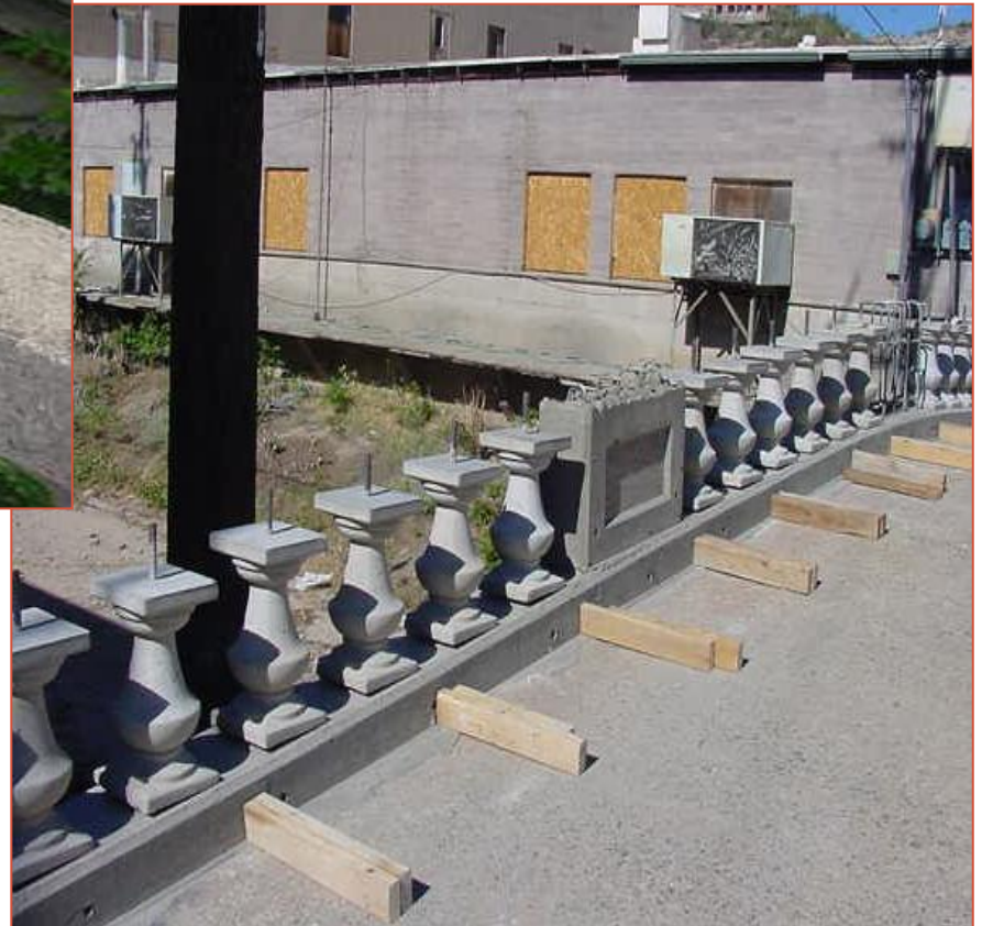
Replaced barrier rail with near replica of historic railing
