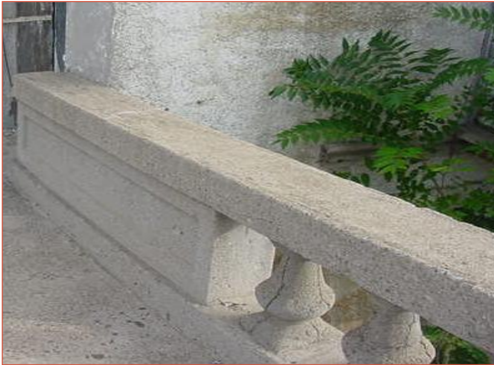
Deteriorated barrier rail in need of repair
