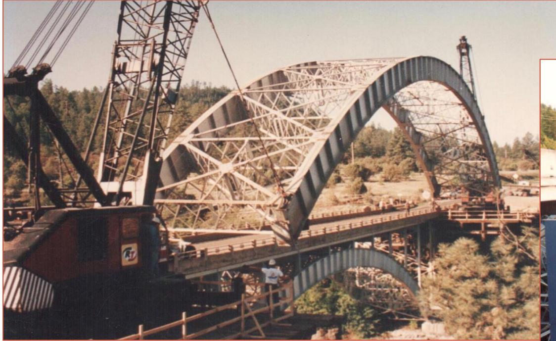
Crane unloading steel arches from Corduroy Creek Bridge
