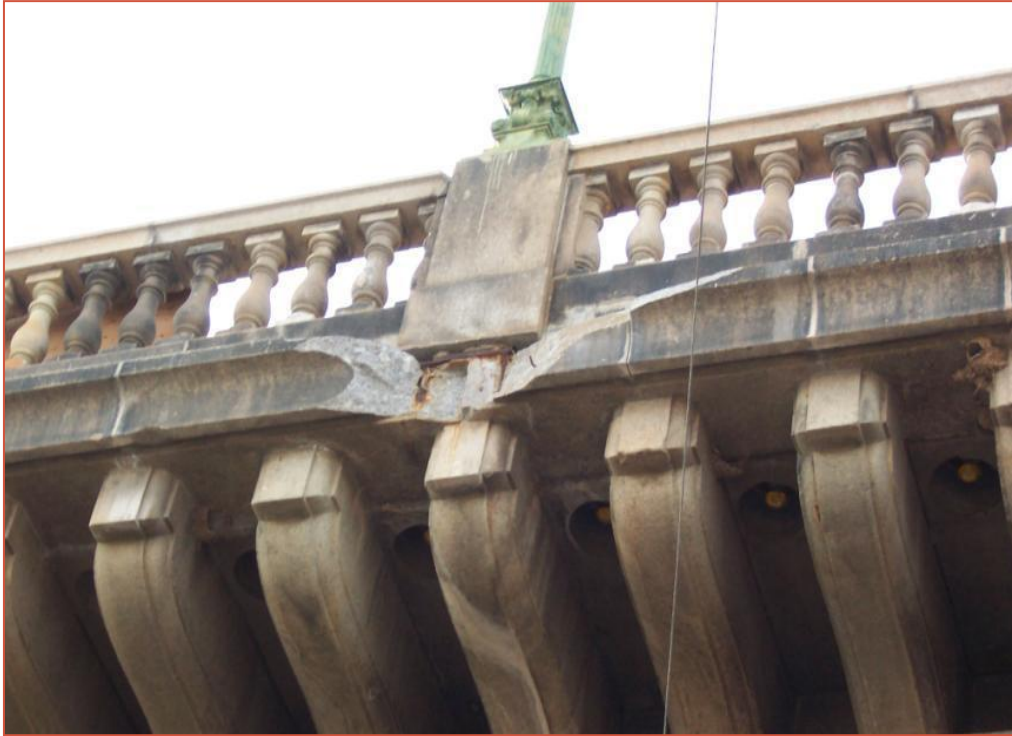
Coping stone cracking at each lamp post
