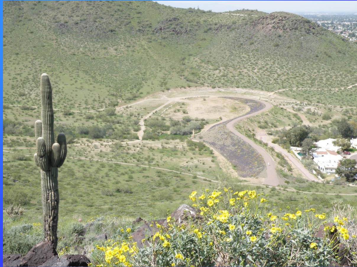
Detention Dam No. 7
