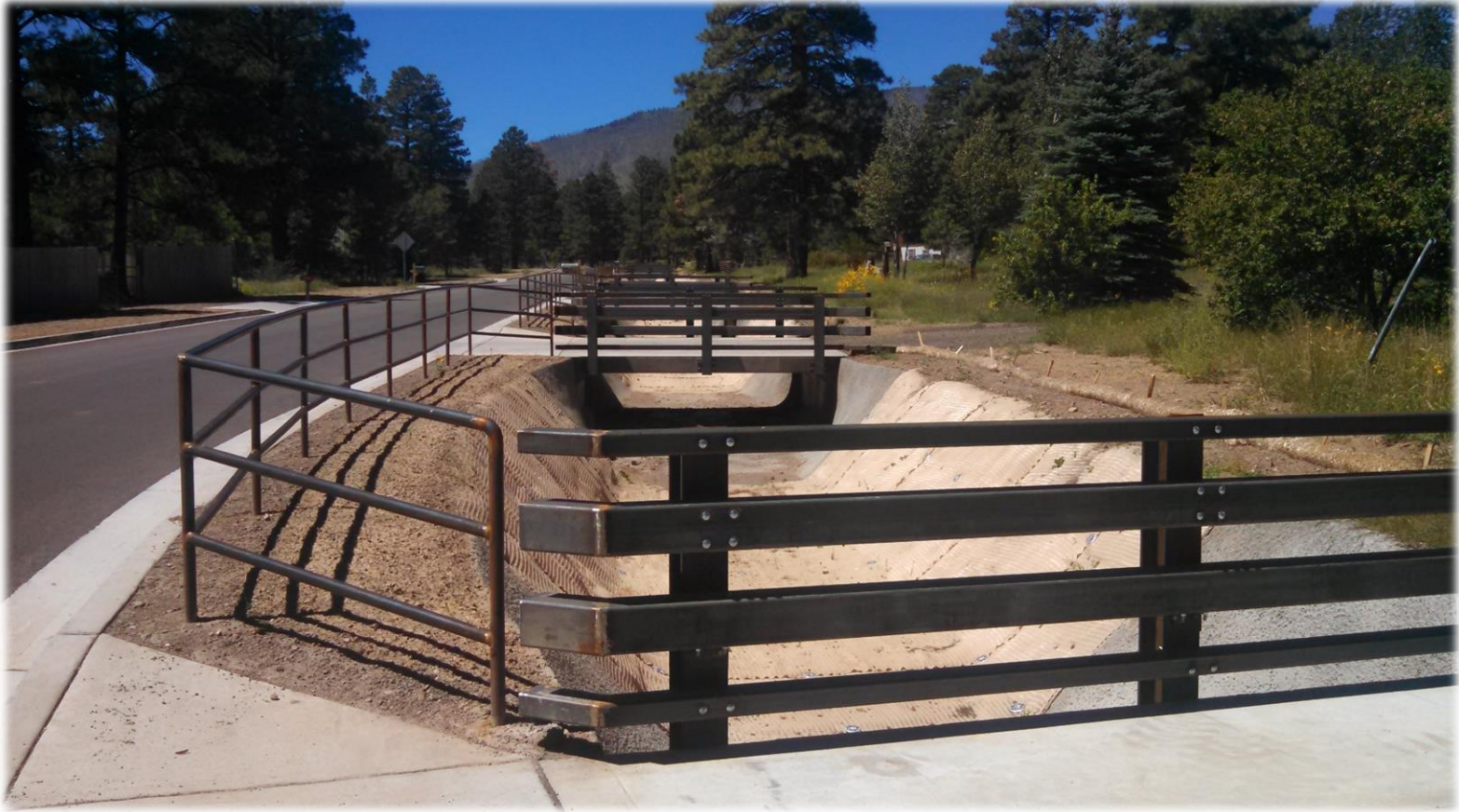
Typical Neighborhood Improvement – Driveway Box Culverts and TRM Channel
