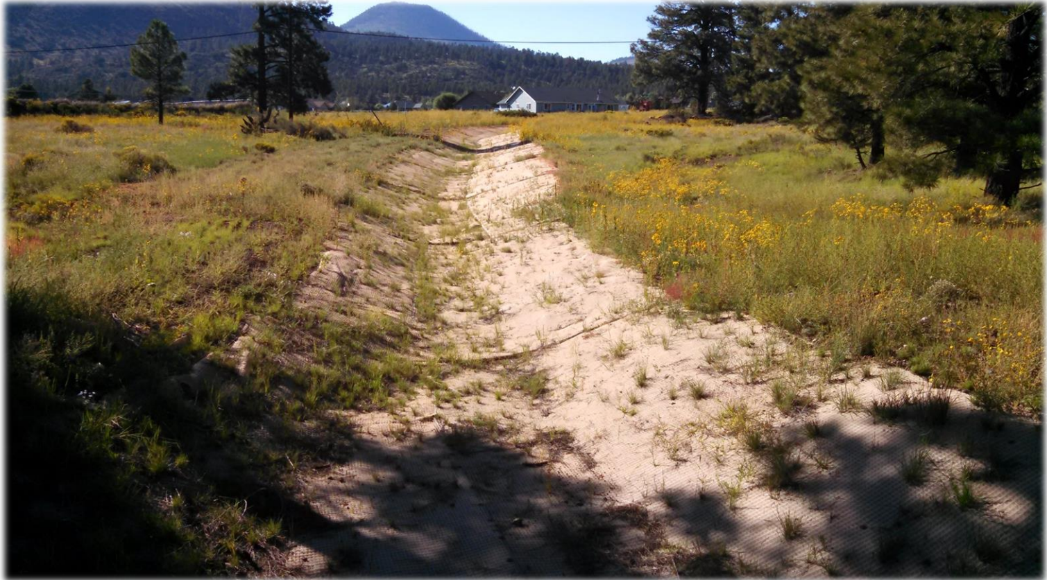
TRM Channel ~ 1 year after construction
