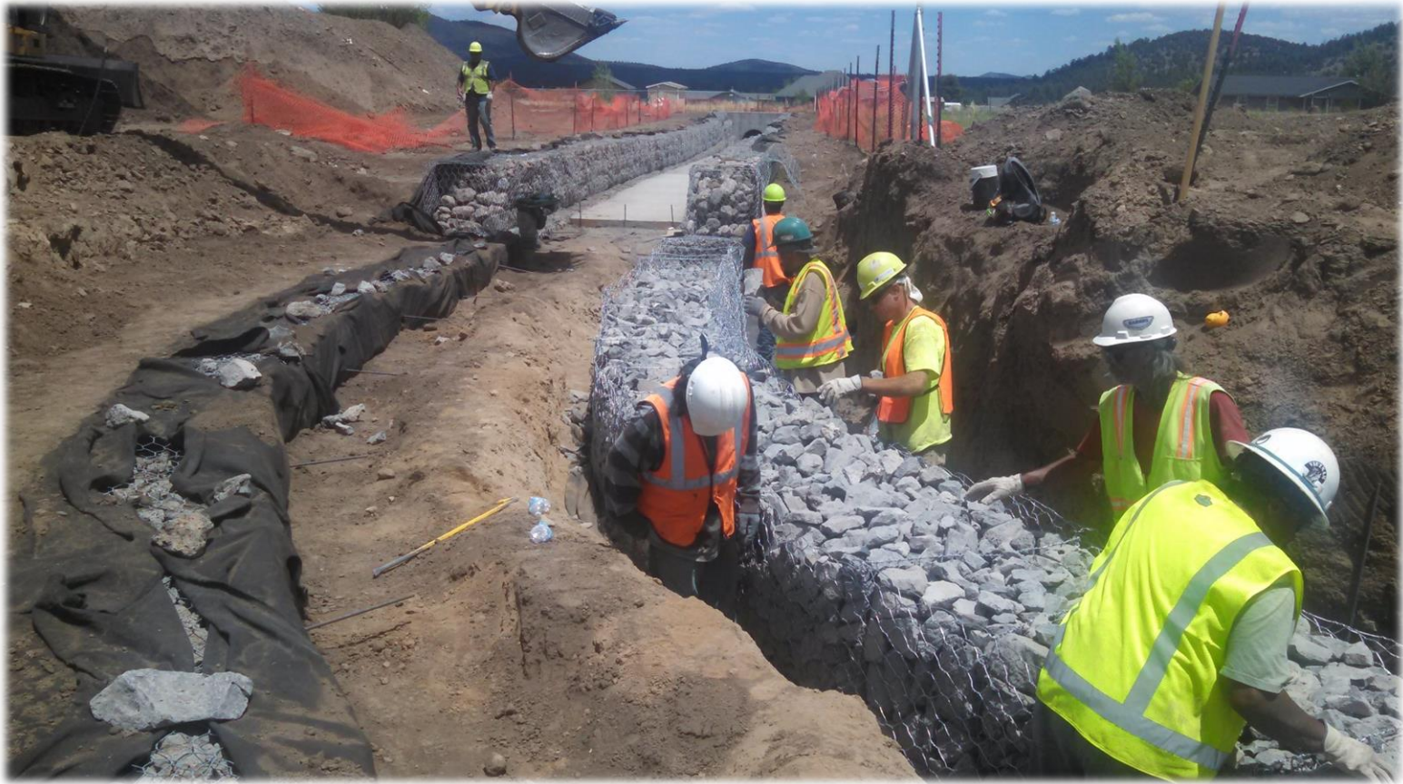
Typical Neighborhood Improvement - Gabion Channel with a Concrete Bottom
