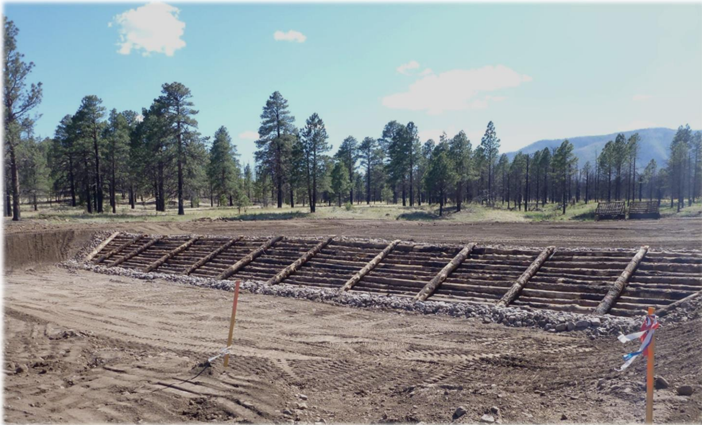
Terminal Trench – Constructed with Forest materials
