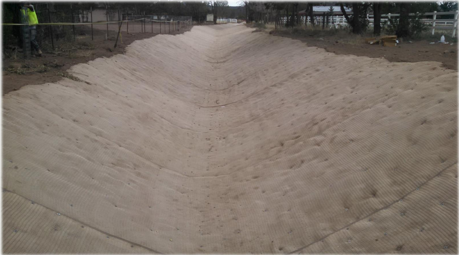
Typical Neighborhood Improvement – Turf Reinforcement Mat (TRM) Channel
