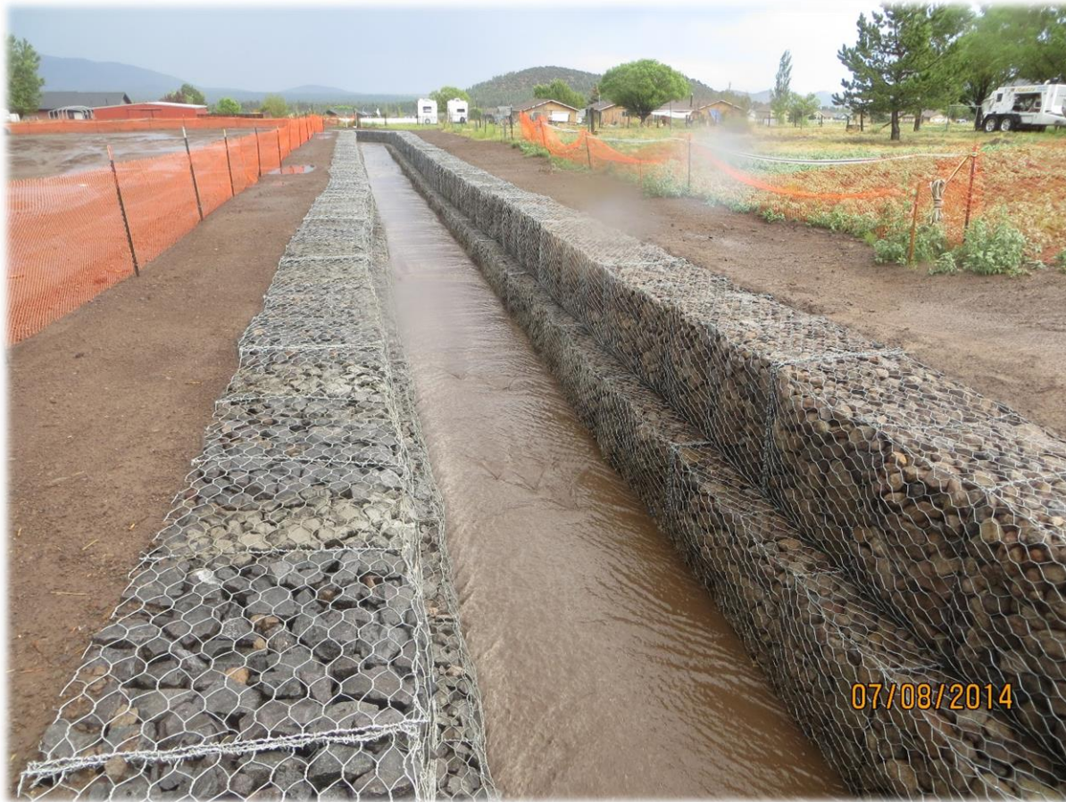
Typical Neighborhood Improvement - Gabion Channel with a Concrete Bottom
