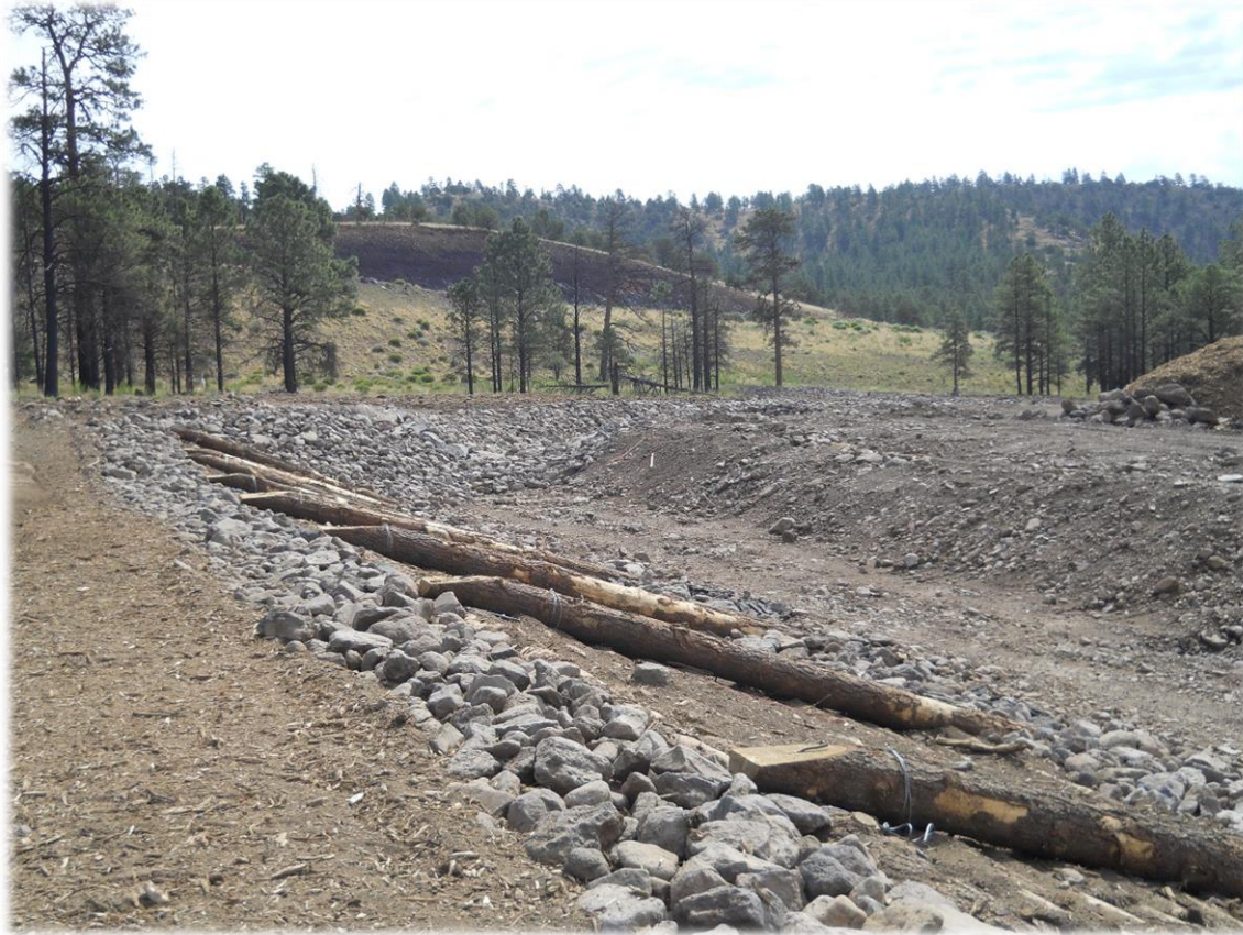
Transition Channel exiting the Terminal Trench
